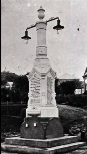
August 1905 Crn Crown Street and Crown Lane, Wollongong
